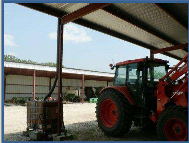
225' x 25' 3 sided metal building for large equipment and hay storage
